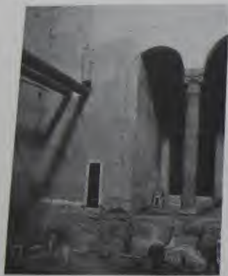
The 4th-5th century brickwork remains of piers, walls and of oratory along the eastern transept.
